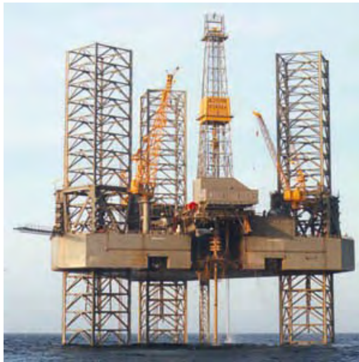
Figure 2.2 Gorilla Class Jackup Rig (courtesy of Rowan)
