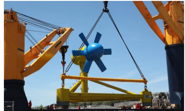
FIGURE 37 - TURBINE-FOUNDATION ASSEMBLING AND OFFLOADING (SOURCE: SABELLA-D10.BZH)
