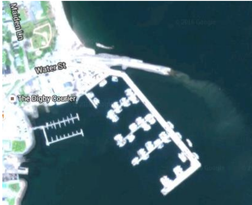
FIGURE 12 – ARIAL VIEW OF FISHERMAN'S WHARF IN DIGBY (IMAGE EXTRACTED FROM GOOGLE MAPS, JUNE 20, 2016)
