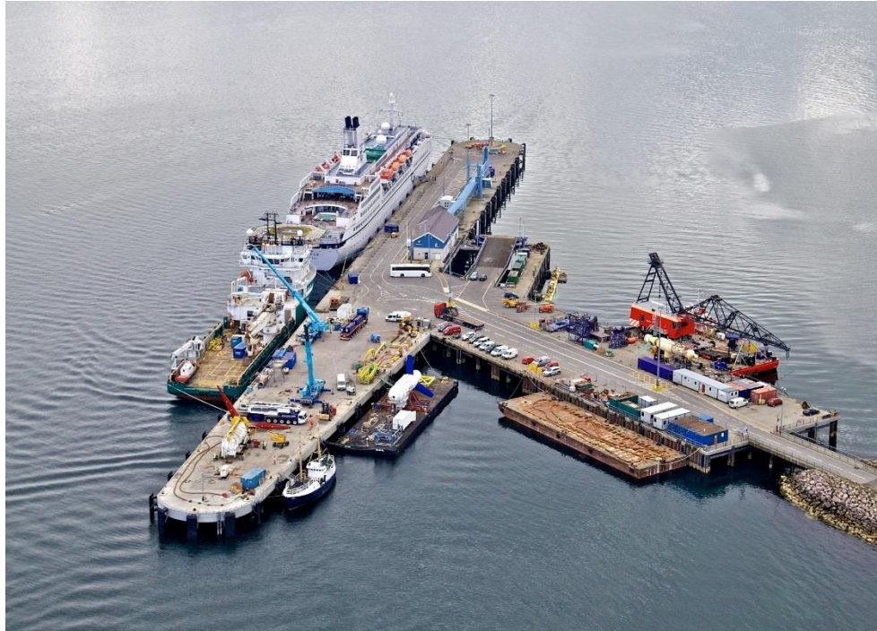
FIGURE 24 - HATSTON PIER UPGRADED (SOURCE: ORKNEY.GOV.UK)
