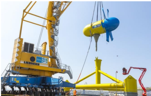
FIGURE 37 - TURBINE-FOUNDATION ASSEMBLING AND OFFLOADING (SOURCE: SABELLA-D10.BZH)
