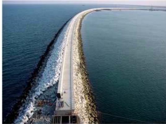
FIGURE 3.8 Breakwater Under Construction with Concrete Armour Units (courtesy Baird & Assoc.)
