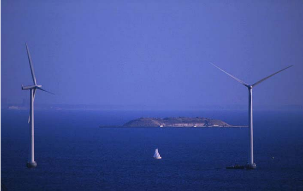
FIGURE 3.2 Photograph of Existing Offshore Wind Turbine in Denmark (courtesy www.windpower.org)
