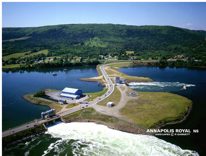
FIGURE 4.9 Annapolis Royal Generating Station
