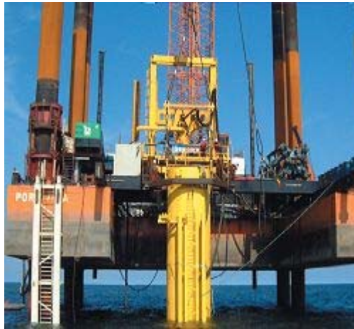
FIGURE 3.13 Installation of a Monopile Using a Jack-up Rig (courtesy UK Seacore)
