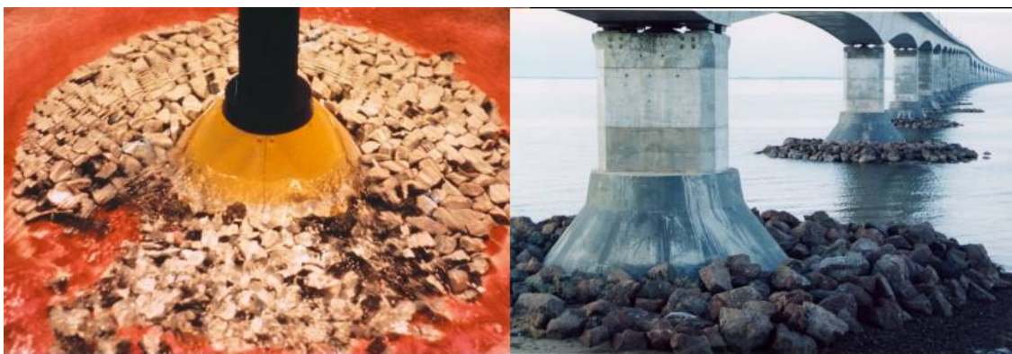
FIGURE 3.14 Physical Model (left) and Installed Scour Protection (right) for the Confederation Bridge (Courtesy Baird & Associates)
