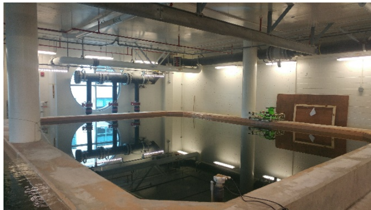
Figure 3: Ballast tank used for testing
