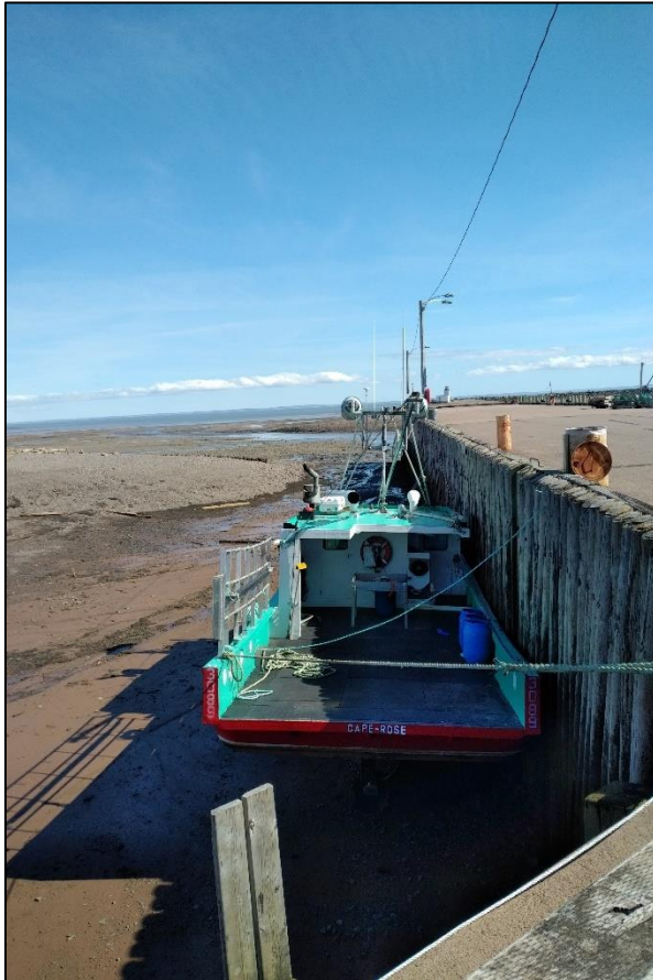
FIGURE 19: PARRSBORO WHARF EAST FACE
