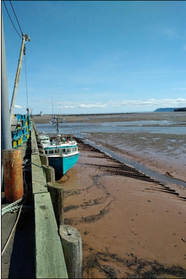
FIGURE 17: PARRSBORO WHARF - WEST FACE & CRIB
