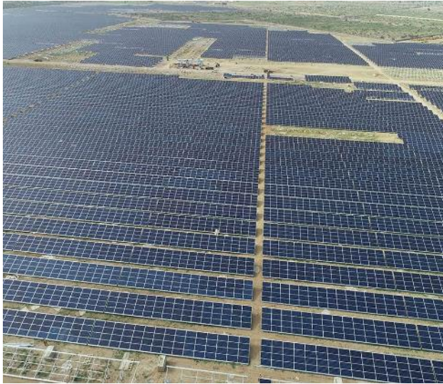
Bhadla Solar Plant, India – 2 245 MW Source: T&D World
