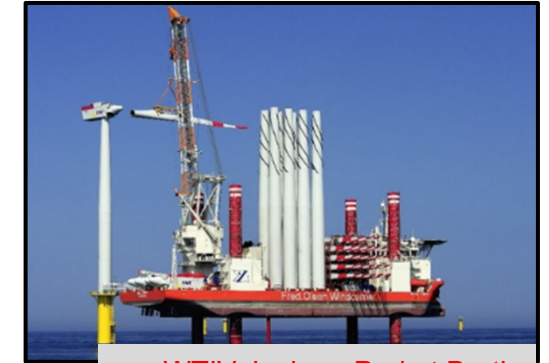
WTIV Jack up Pad at Berth
